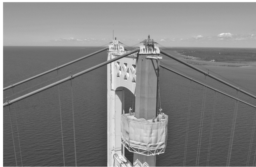
The Mackinac Bridge tower painting project, now entering its fourth and final year, has won a third national award for the movable scaffold platforms designed by Ruby+Associates. Courtesy photo.
